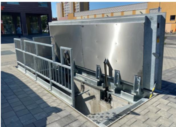
Hydraulic escape hatch with collapse protection, Berlin
