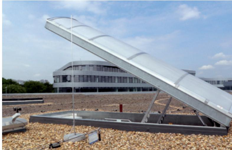
Small escape hatch that can be opened by hand, Cologne
