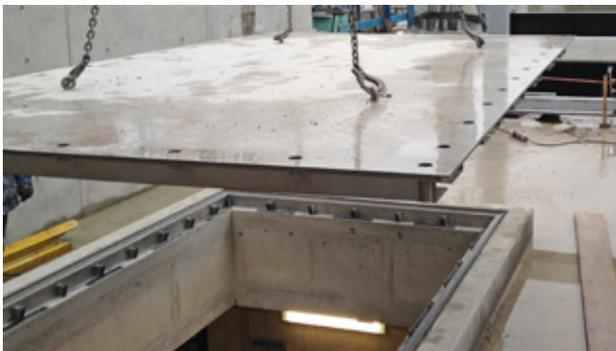
View from below of a floodproof cover on an assembly opening, power plant on the river Danube near Augsburg
