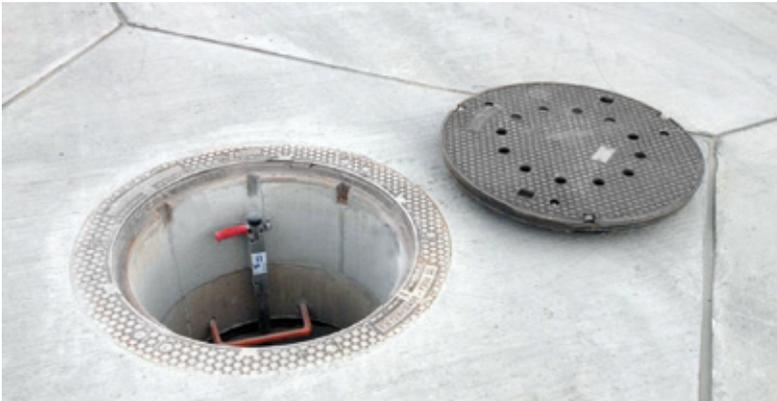
Cast-iron cover with screw-in locking lever fastenings, a load class of F 900 and a clear opening of 800 mm
