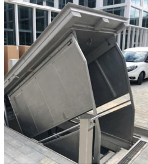
Hydraulic escape hatch cover, Stuttgart
