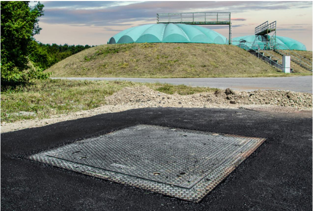
Surface-water-tight cast-iron cover, load class D 400, Munich
