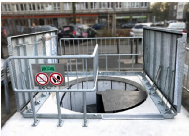
Escape hatch cover, safe to walk on, can be operated manually, Essen
