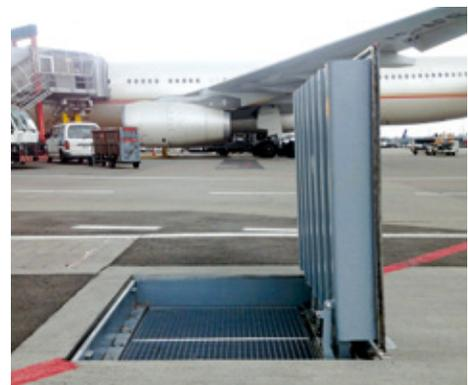
Access and assembly opening, load class F 900
