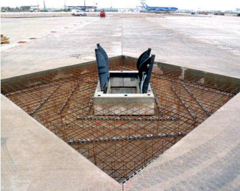
Prefabricated triangular cable shaft covers with a height-adjustable reinforced concrete frame and a load class of F 900, Frankfurt
