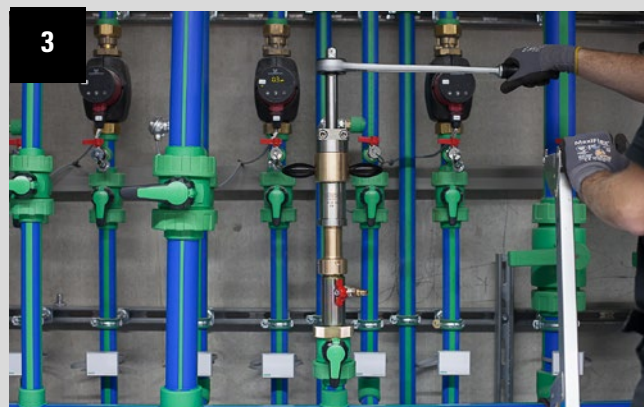
3. Start of the drilling process
