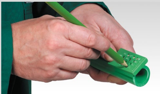
Marking of the welding depth
