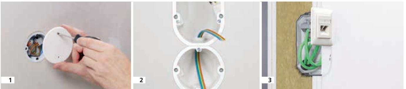
**1** For use as a junction box when fitted with a fire-protection cover.
