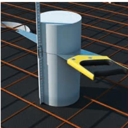
Shorten the formwork unit to match the ceiling thickness.
