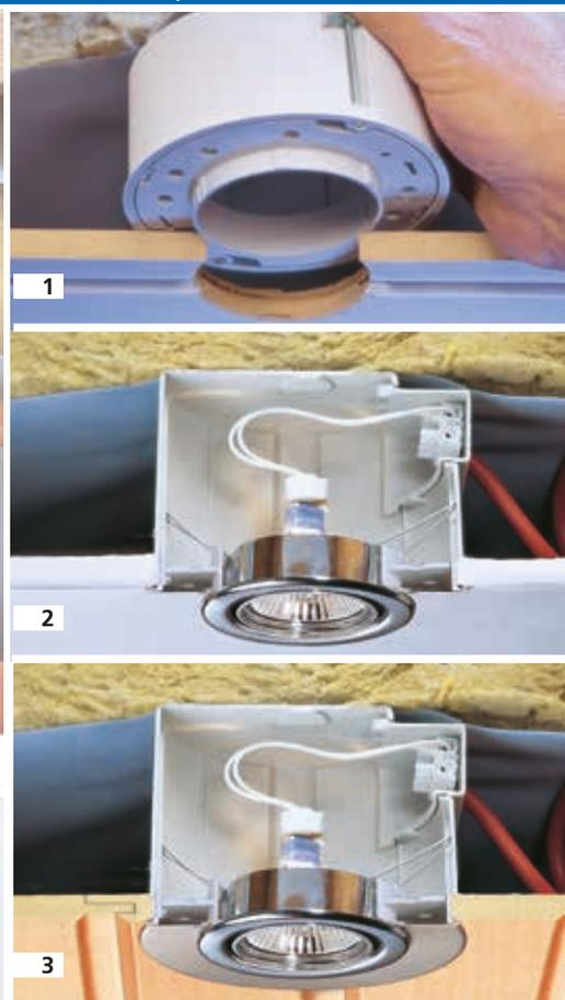
Latent fire risk caused by temperatures of more than 200°C from halogen lamps can occur very quickly. The ThermoX® installation housing prevents the transfer of extreme heat development to all the surrounding materials.
