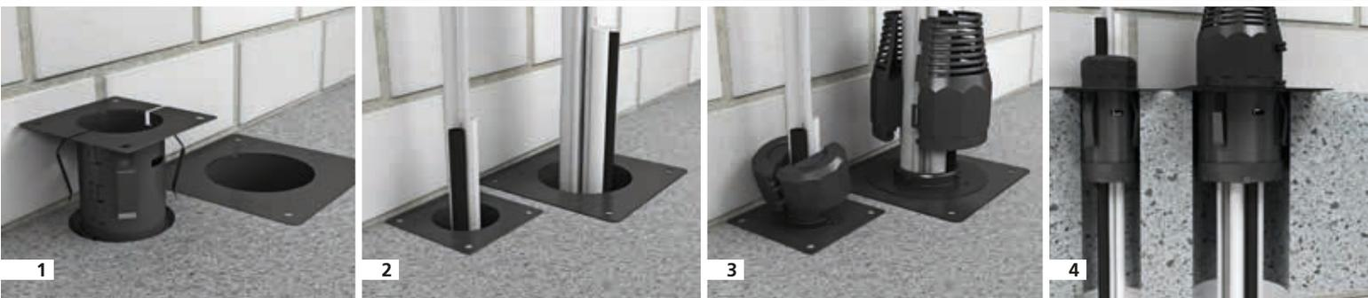
Installation takes place easily and quickly from the ceiling upper surface. The ceiling seal system can also be retrofitted around existing cables and conduits. Non-destructive later fitting of additional cables up to full population is possible at any time.
