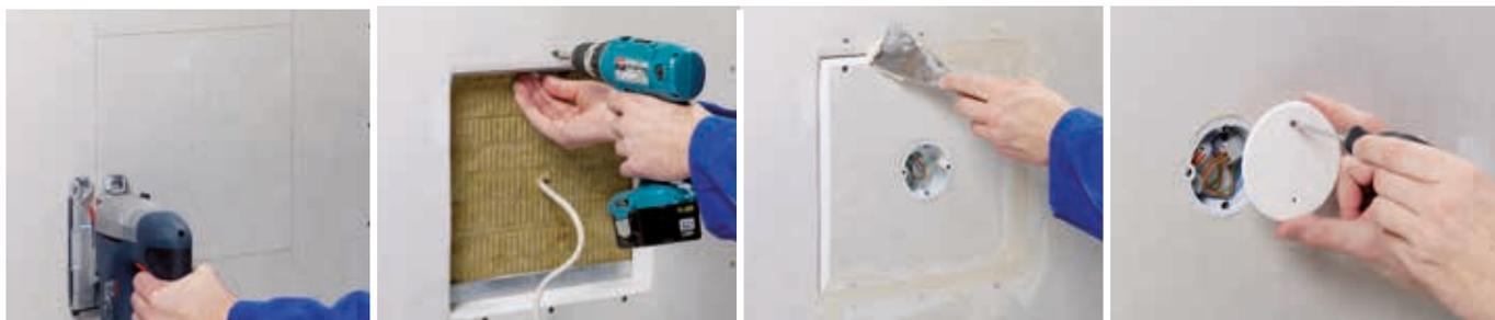
Depending on the required period of fire resistance, the component opening must be backed with a different type of mineral wool (I30 without insulation, I60 insulation material DIN 4102-17, I90 Rockwool/Termarock 100). To fit the mineral wool, a cut-out of at least 300 x 300 mm is needed in order to create space for perfect installation.
