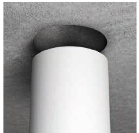
After striking the formwork, remove the formwork unit without residue from the component opening.
