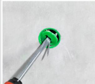
After striking the formwork, use a screwdriver for fast, easy opening of the plaster skin.
