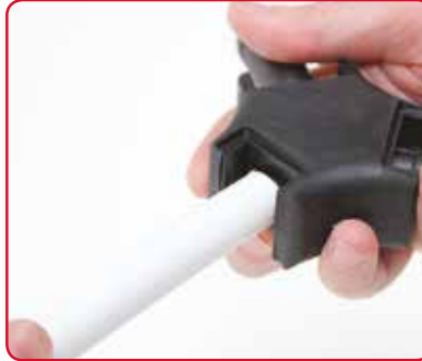
2. Bevel the cut end of the pipe.
